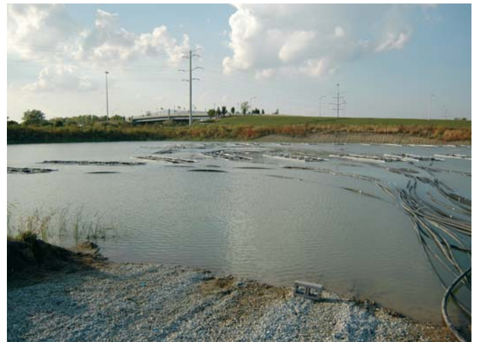
Loop Coils prepared for submersion into the pond.
