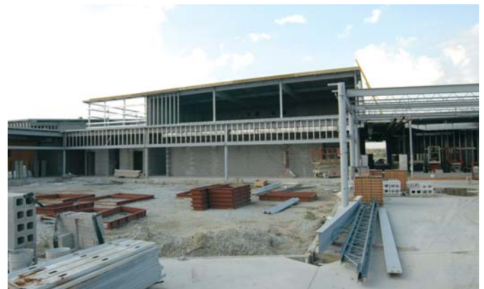
Construction in progress on the school grounds.
