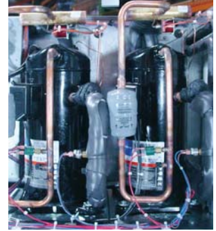
Copeland Scroll compressors (dual circuited on 8 ton and larger)
